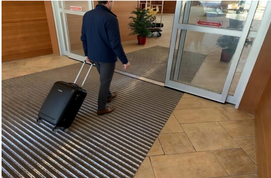
Completed entrance mat at the main entrance of the private airport.
