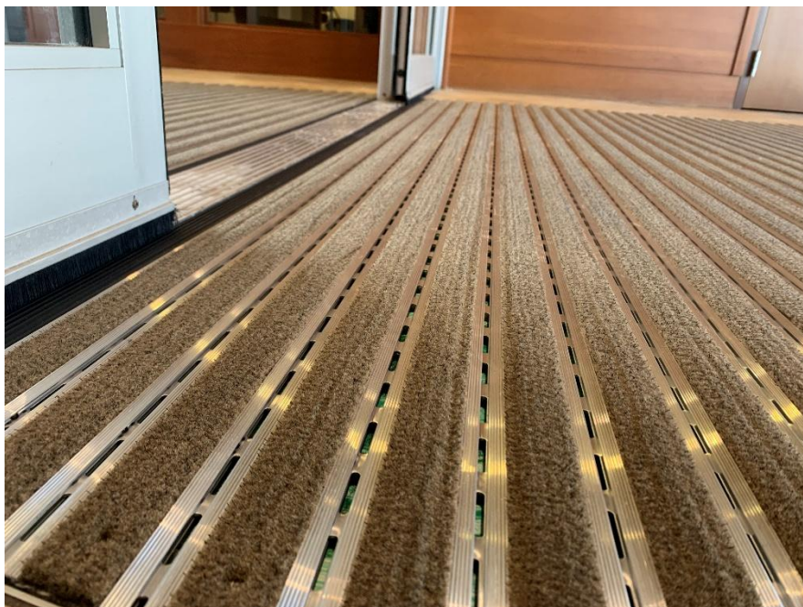
Close up view of the aluminum entrance rails for this project.
