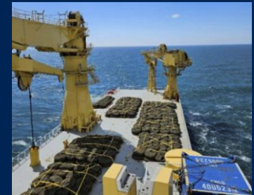
Third party vessel – Filter bag installation
