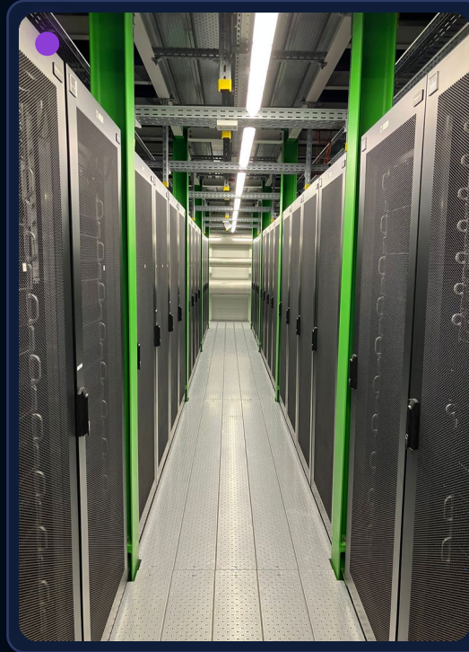
Cold-aisle containment
