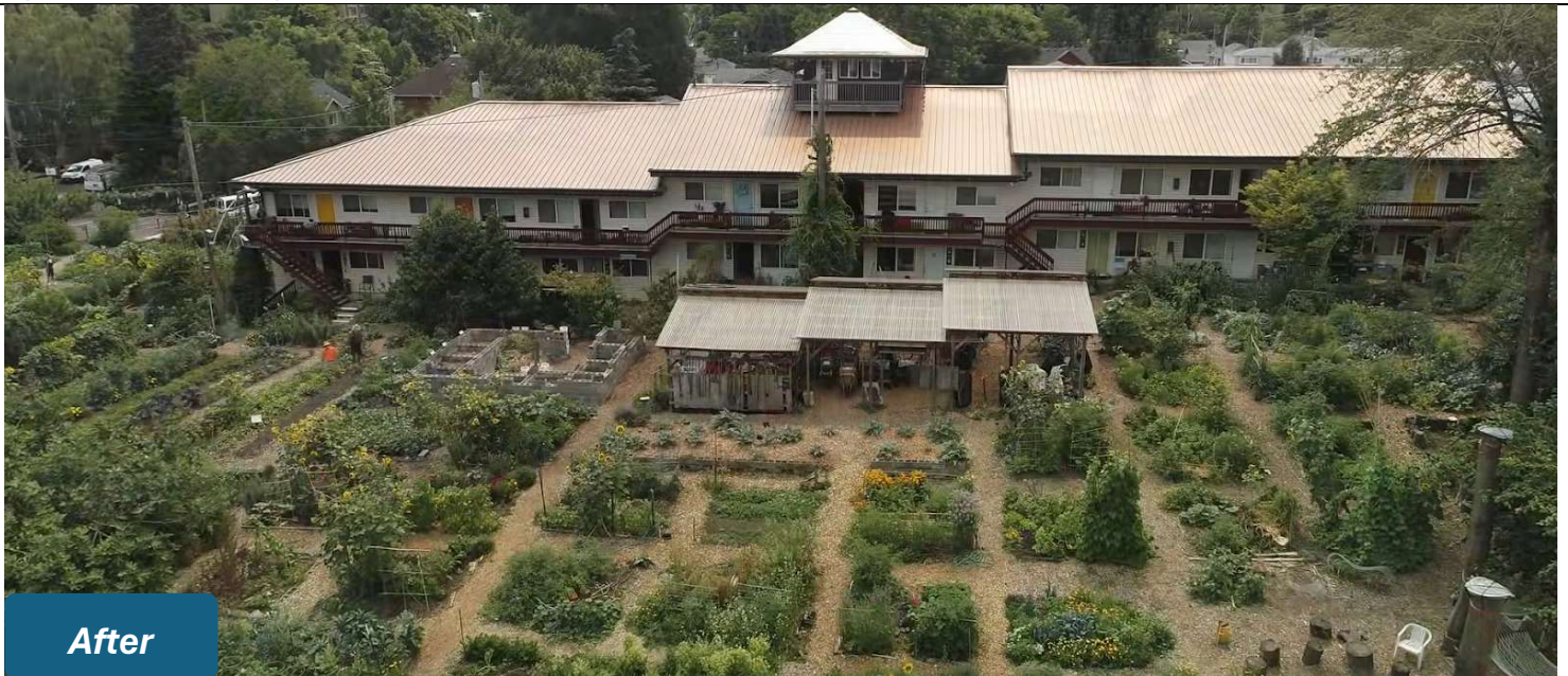
Figure 8. Kailash Ecovillage after renovations iv
