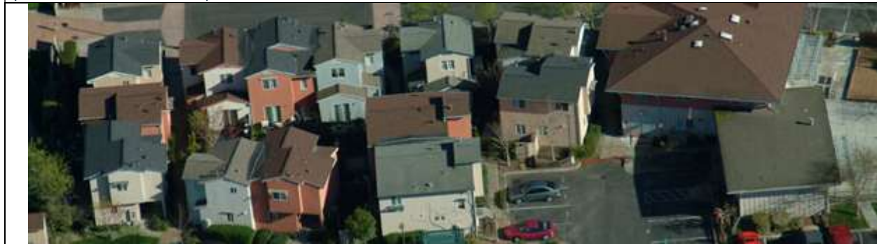
Figure 6. Aerial view of Round Walk Village
