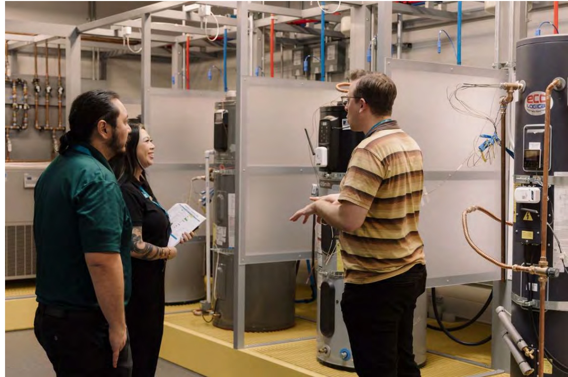
Heat Pump Water Heater Lab
