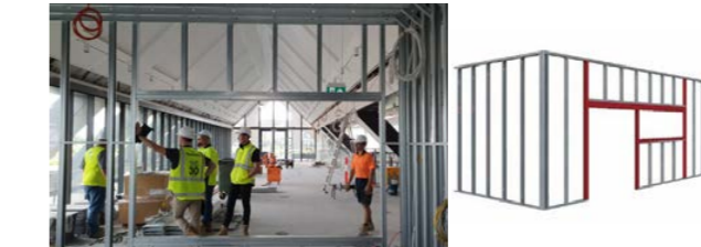
HEDA TOUGH WALL SYSTEM The fast and easy way of creating openings in internal and external walls.
