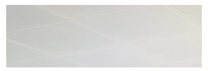
SAS130 offers either a flush (Alugrid) or tegular (Tee Grid) finish metal ceiling, depending on aesthetic preference. Lay-in tiles are quick to mount and dismount offering simple access to the ceiling void.
