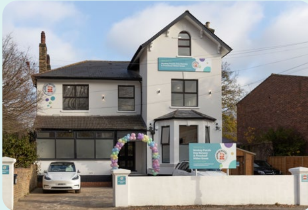
Example of building frontage with parking
