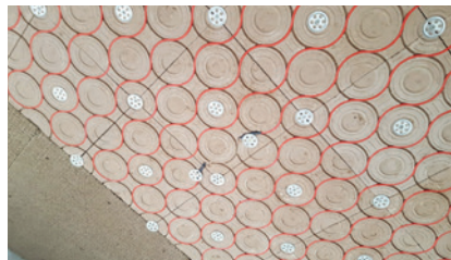
High performance clay modules with clay compensation panels & inserted heating cable
