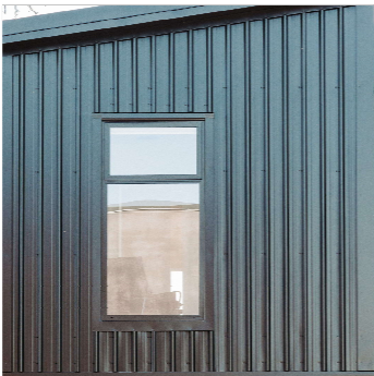
Metal cladding - Vertically fixed Colorsteel cladding- trapezoidal
