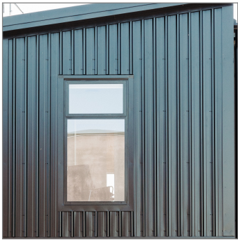
Metal cladding - Vertically fixed Colorsteel cladding- trapezoidal
