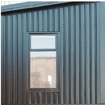
Metal cladding - Vertically fixed Colorsteel cladding- trapezoidal
