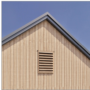
Architectural Feature - Decorative Cedar Louvre
