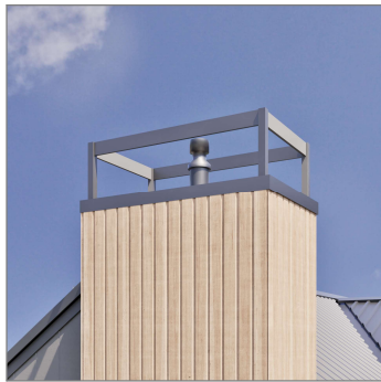
Architectural Feature - Boxed Chimney cowl
