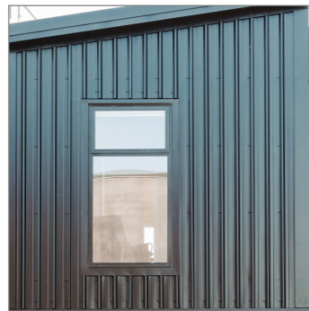
Metal cladding - Vertically fixed Colorsteel cladding- trapezoidal
