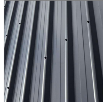
Metal cladding - Vertically fixed trapezoidal
