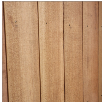
Natural cladding - Selected Vertical Cedar w/board cladding
