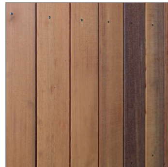
Natural cladding - Selected Vertical Timber w/board cladding
