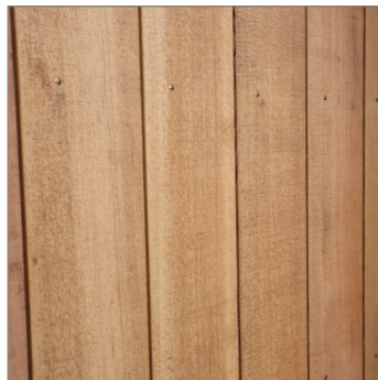
Natural cladding -Selected Vertical Cedar w/board cladding
