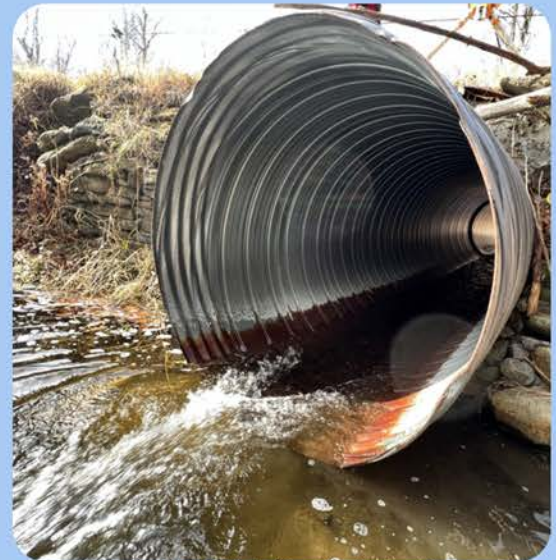
North Branch Silver Brook culvert
