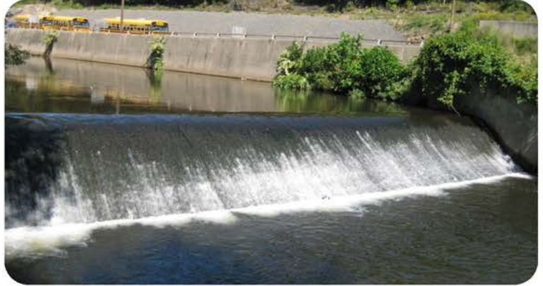
Princeton Hydro is working with CT DEEP and DOT to complete plans for the removal of Middle Street Dam in Bristol, CT
