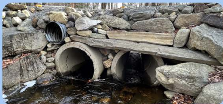
Shales Brook culverts
