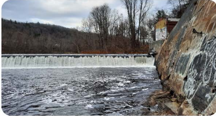
CT DEEP is coordinating the removal of Lower Collinsville Dam to improve fish passage and to create safe public access on the river
