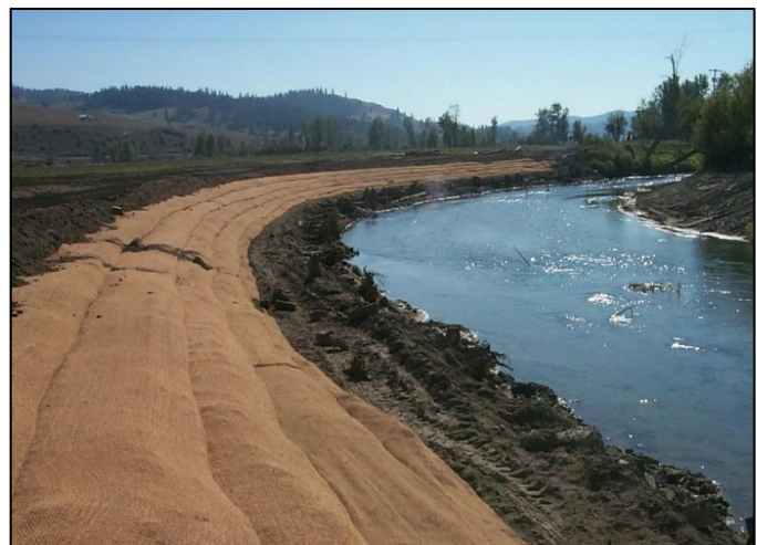
Re-sloped bank with stabilized toe
