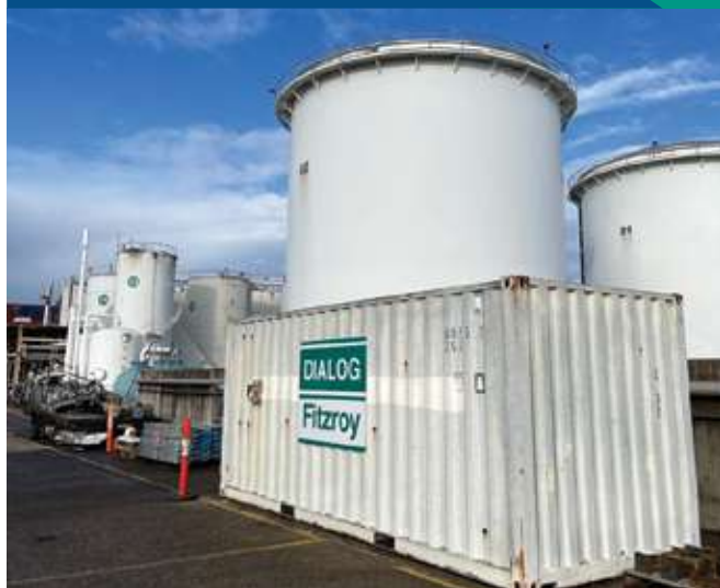
Tank inspection and maintenance for Quantem, Australia
