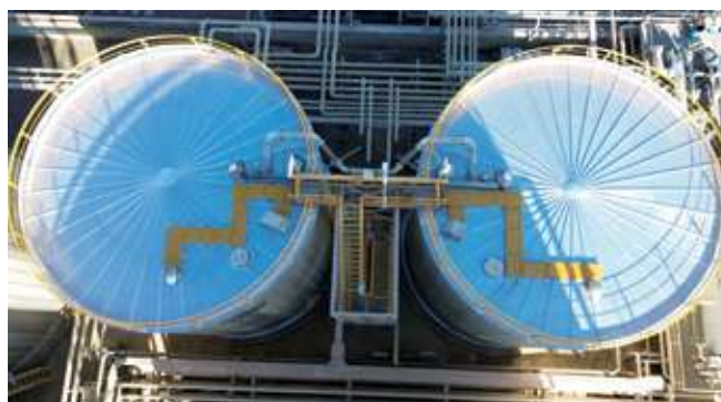
Tank turnarounds for Puma Energy, Townsville, Australia
