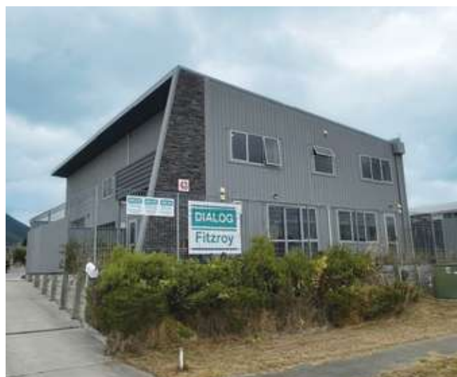
New Office in Taupo, New Zealand
