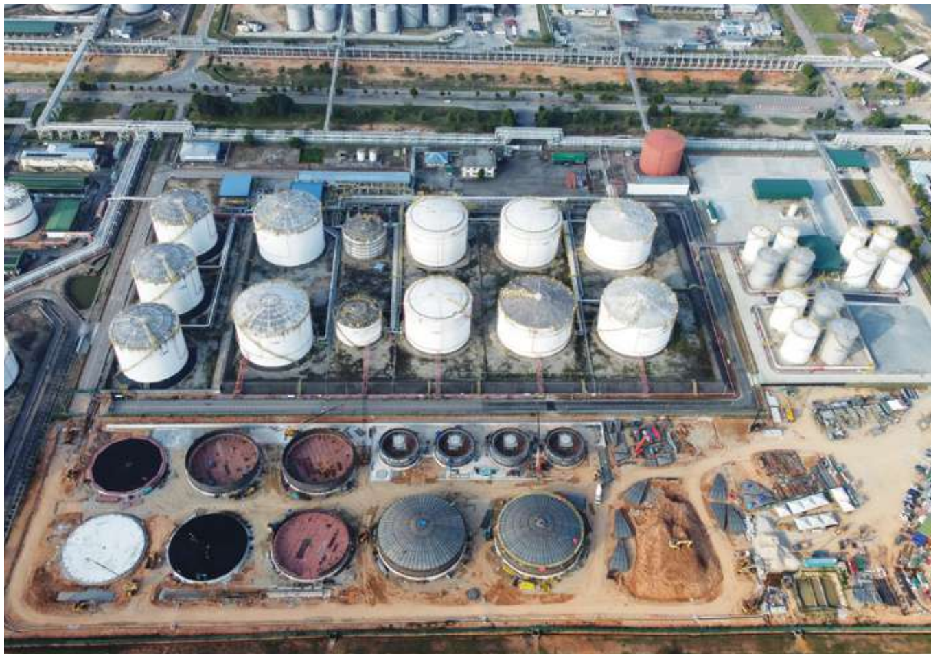
The first and second phase of storage facilities for renewable fuel products, DIALOG Terminals Langsat 3
