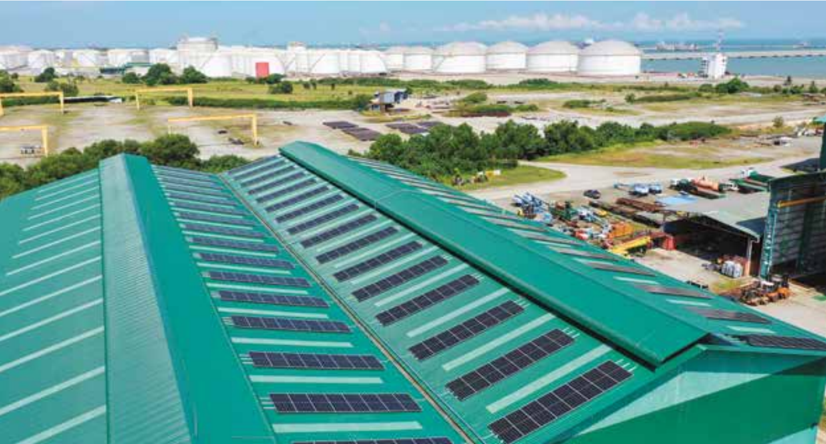
Solar panel installed at DIALOG's fabrication yard in Pengerang, Johor
