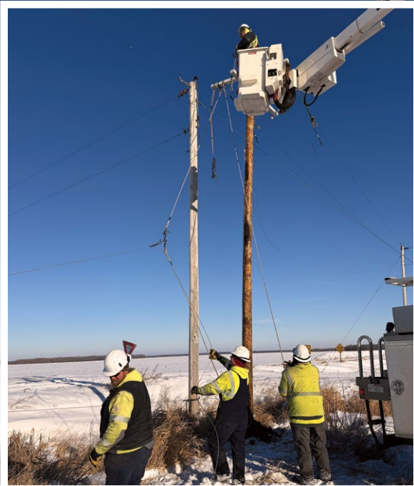
REC linemen (left to right) Chad Johnson, Connor Eidsmoe, Ross Nelson and Justin Olson (in the bucket) work on a single-phase pole changeout in Moose Township north of Badger.
