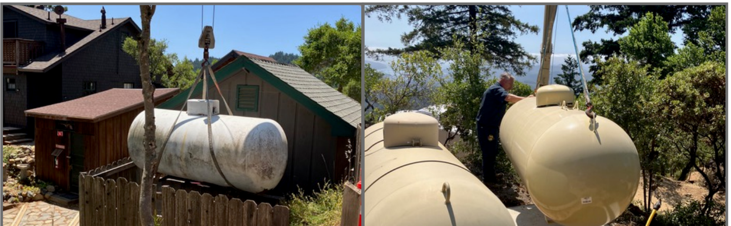
Relocating West Point Inn's 500 gallon propane tank Photos submitted by Don Keeley
