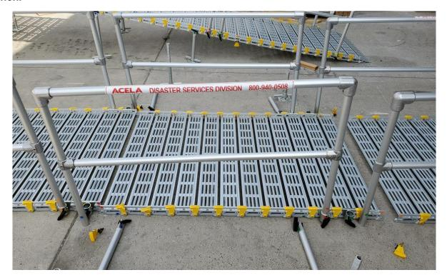
Check that all bolts and hand screws are tight, that all detent pins are secured in place, that ratchet strap (ramp to trailer) is tight and all legs are adjusted properly.
