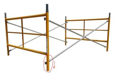
Insert the level jacks into the bottom of the scaffold panels, but do not start leveling yet:
