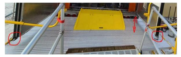
Once the desired height is set and platform is level, add the corner posts to the corners of the scaffold closest to the trailer. Also add the P-Poles to the corners of scaffold furthest away from the trailer, ensuring that the P-shaped protrusions face each other and are fully extended:
