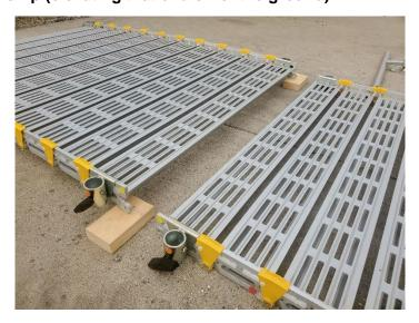
Carefully unroll the next ramp section (indicated by color coded dots on the side of the ramp – Yellow (towards first section) and Red (towards street end of ramp). Marry the Yellow end of the second ramp to the Yellow end of the first ramp (resting on 2x4 lumber). Insert locking detent pins to secure sections. Make sure detent pins are inserted all the way.
