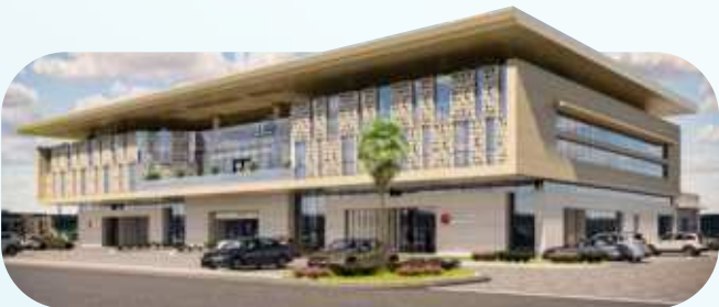
DSFMC Al Hamra, Riyadh
