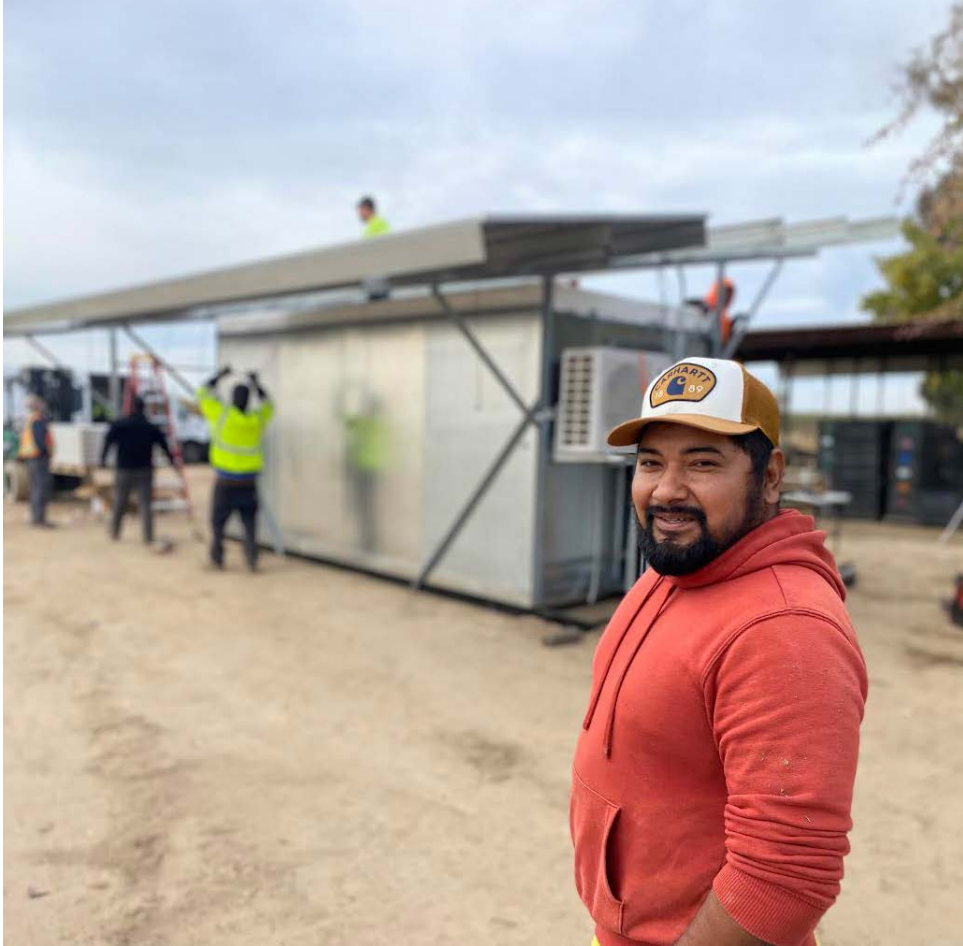
Javier Cruz overseeing the installation of a solar cooler on his farm near Chowchilla.
