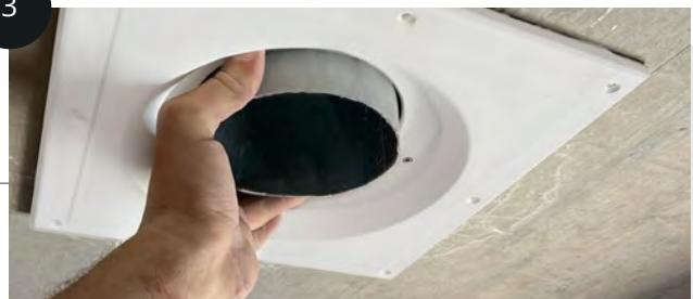
Position the Wallflow element over the duct and adhere it directly to the concrete ceiling using MS Polymer High Tack. Finish the plaster flush with the element.
