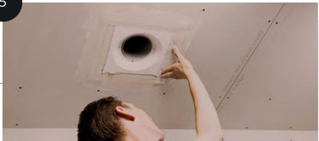
Apply joint tape over all four seams and finish with another layer of fibre-reinforced filler.
