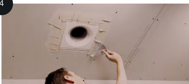
Prepare a fibre-reinforced filler and press enough material into the joints to provide additional strength. Smooth it level with the plasterboard surface.
