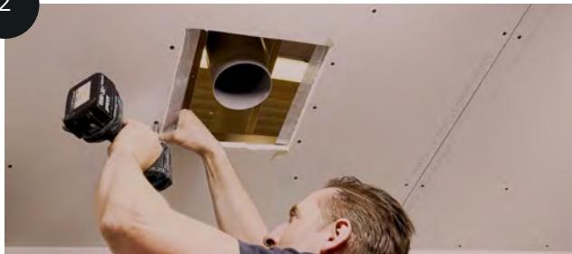
Attach the supplied mounting brackets with the **raised side facing downwards** in the opening.
