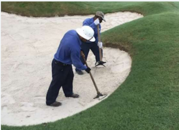
Compacting sand manually
