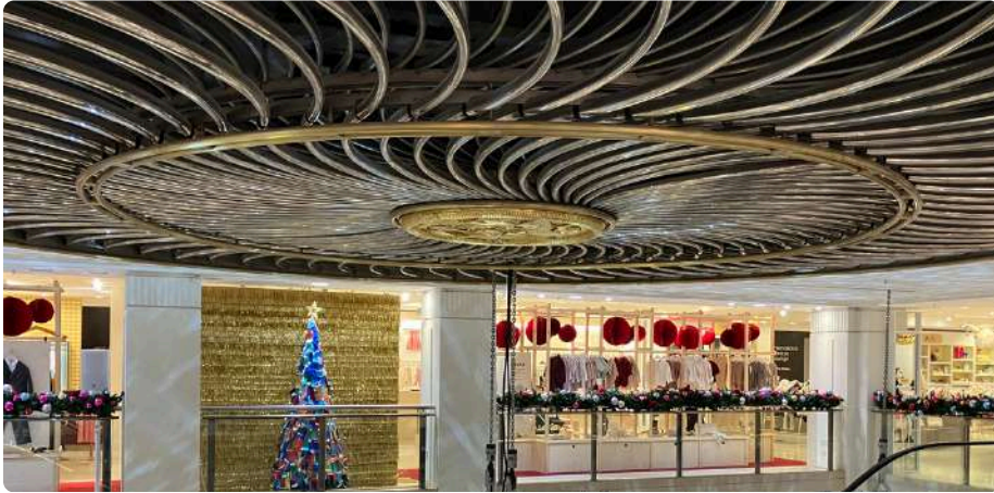
Feature air vent at Selfridges, London (oval tube, stainless steel 316L, 61 x 37 x 2mm)
