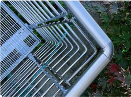
Balcony railing, California (oval tube, stainless steel 316L, 47 x 25 x 2mm with B Plane connectors)
