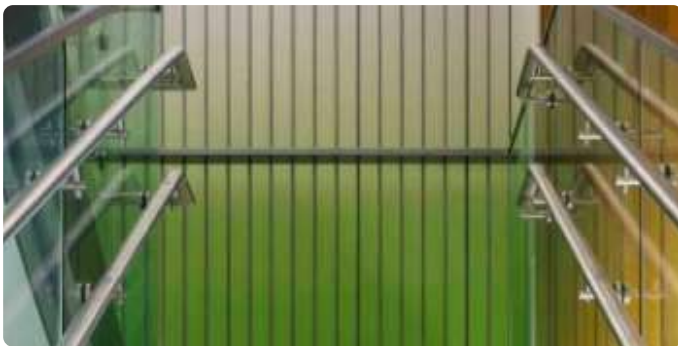
Handrail, 110 William St, NYC (oval tube, stainless steel 304, 47 x 25 x 3mm with A Plane and B Plane connectors)
