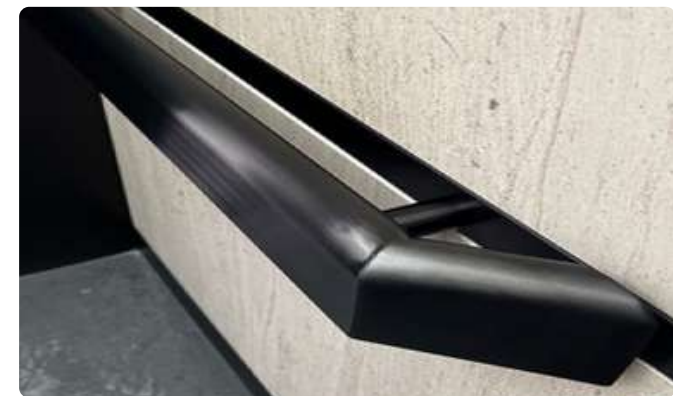
Lift car grab rail (flat-sided oval tube, stainless steel 304, 99 x 38 x 1.5 mm, mitre-cut at 45° then welded without connector)
