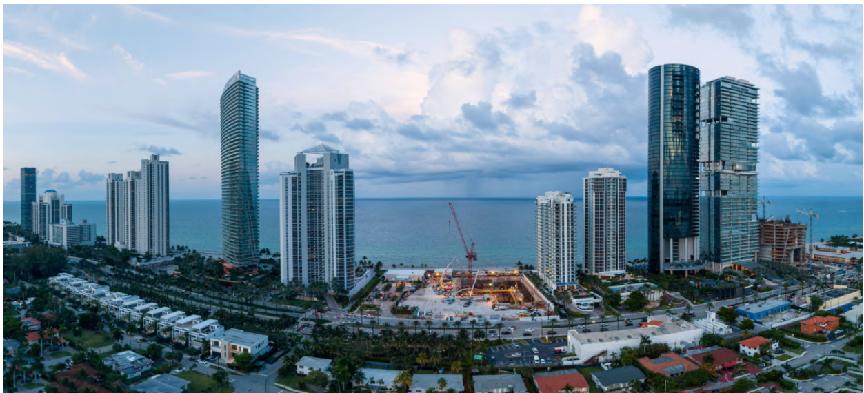
With the Atlantic Ocean in view, Coastal Construction crews complete the South Tower's landmark mat pour at The St. Regis Residences, Sunny Isles Beach, Miami.
