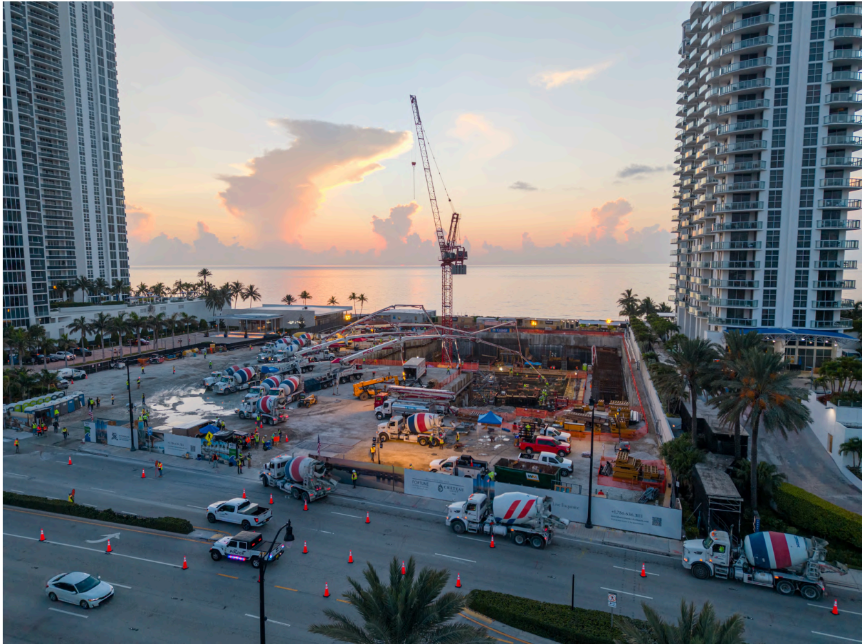
The South Tower's mat pour takes shape, setting the stage for vertical construction this year.
