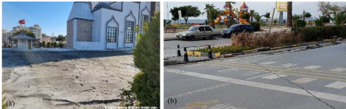
Figure 6. Post-earthquake ground deformations observed near the Nihal Atakaş mosque: (a) sediment ejecta (36.5933N, 36.1574E; photo by Eylem Arslan taken February 14, 2023), and (b) lateral spreading along Atatürk Boulevard (36.5933N, 36.1594E; March 28, 2023).
