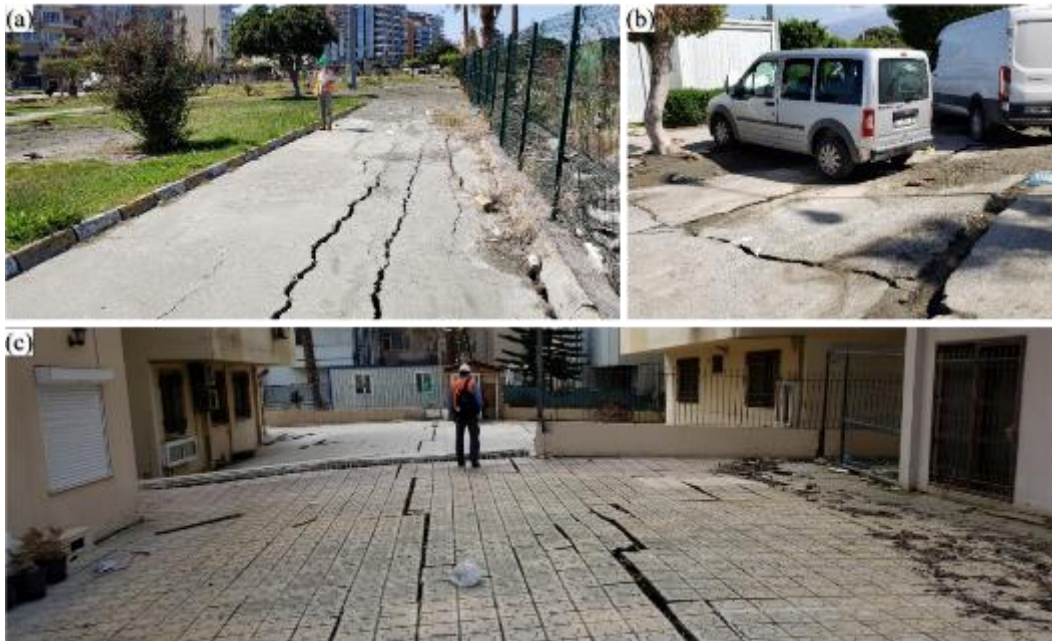
Figure 11. Post-earthquake ground deformations observed in the Çay District: (a) possible sand ejecta and lateral spreading near boat dock (36.5915N, 36.1789E; April 1, 2023), (b) cracks along Atatürk Blvd at the north end of transect LS-5 (36.5908N, 36.1767E; April 1, 2023), and (c) ground deformation and extensional cracks between settled buildings near LS-7 (36.5907N, 36.1792E; March 28, 2023).
