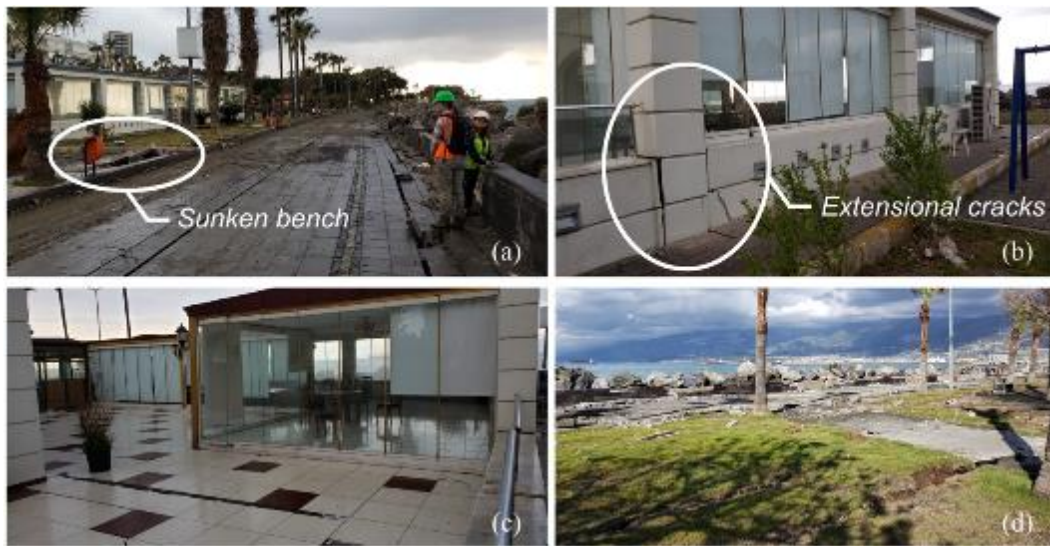
Figure 9. Lateral spreading at the Doğan restaurant and Emekliler park observed on April 1, 2023: (a) sunken park bench and shorefront damage behind Doğan restaurant patio (36.5936N, E36.1674E), (b) patio east exterior wall damage (36.5934N, 36.1672E), (c) patio damage (36.5935N, 36.1671E), and (d) transect LS-4 in Emekliler park (36.5930N, 36.1687E).
