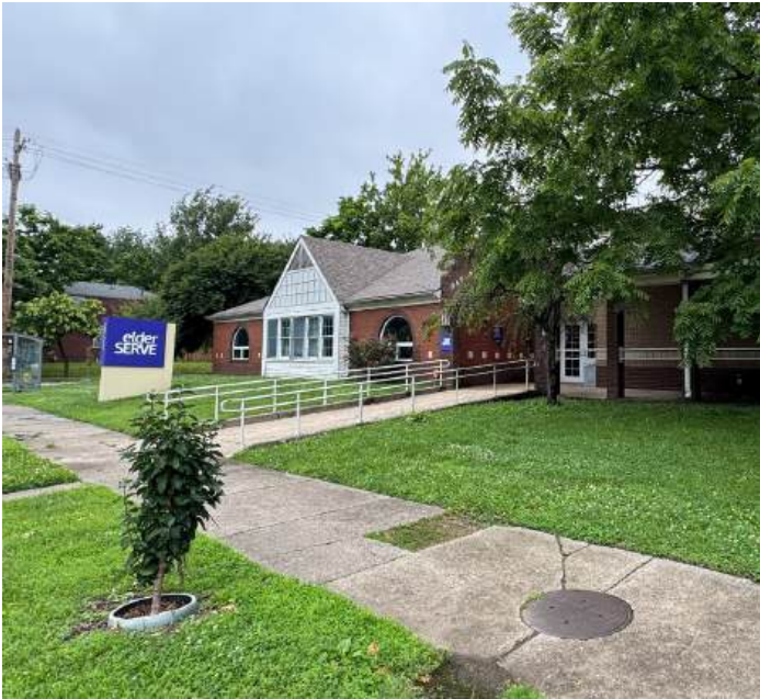
■ The ElderServe building at Magazine Street and 28th Street — Photo taken by the project team
