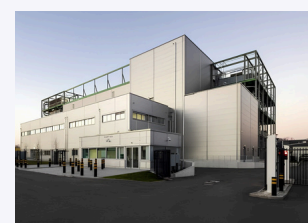
Google Data Center Hanau, Germany
