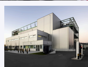
Google Data Center Hanau, Germany
