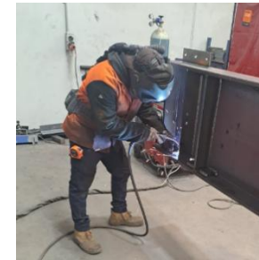
In-house fabrication, welding and paintwork
