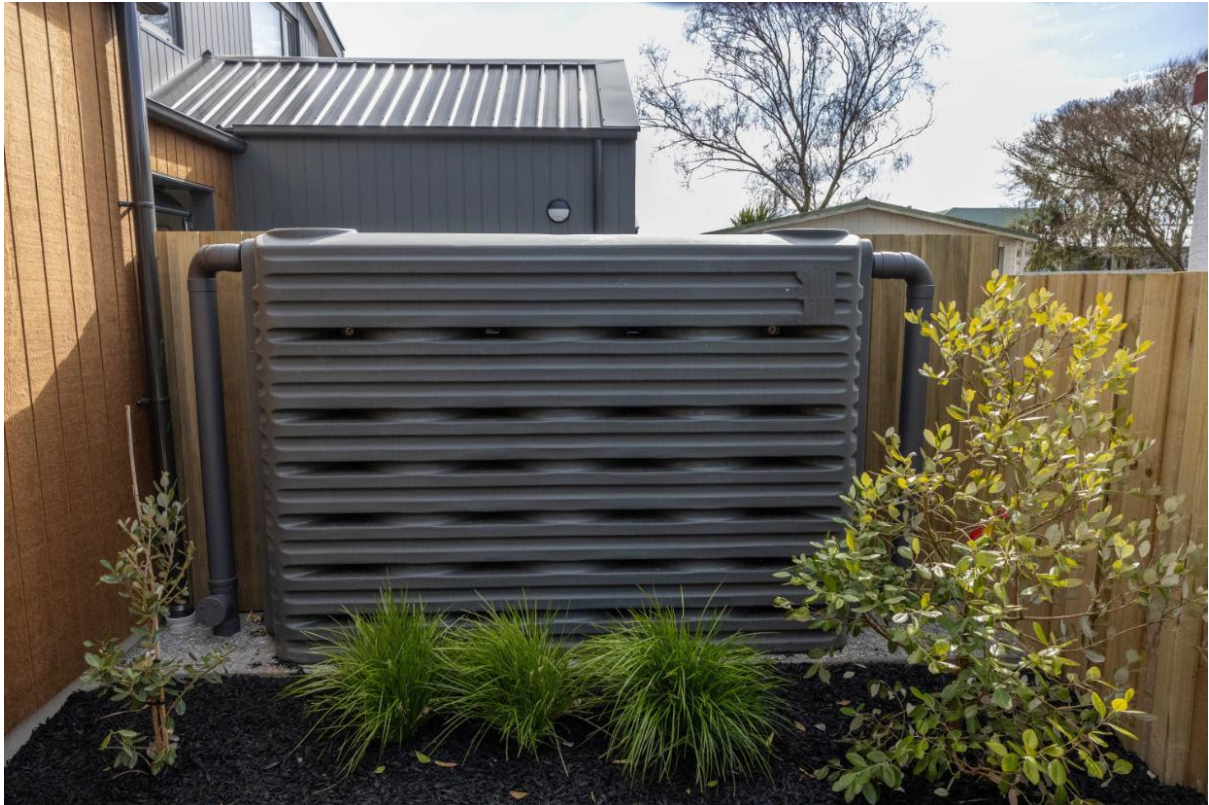
A water tank which collects water from the roof.
