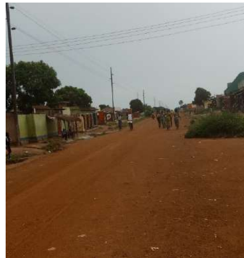
Kashikishi - Lunchinda after grading
