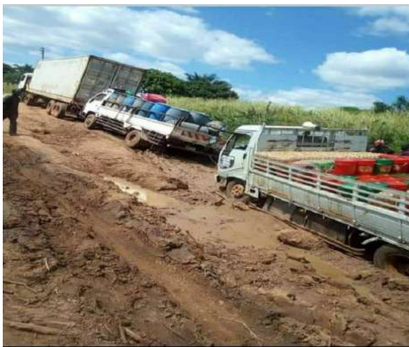
Kashikishi - Lunchinda Road(D79) During Rainy season Source: Chiengge Town Council (2023)
