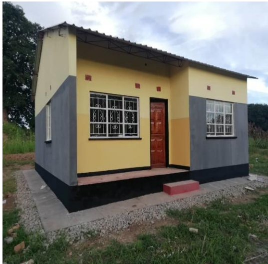
Figure 10: Examples of permanent structures built in rural areas (MTC Public Relations- 2022)
