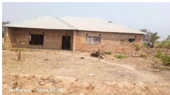
(b) unfinished house built with mold bricks.
