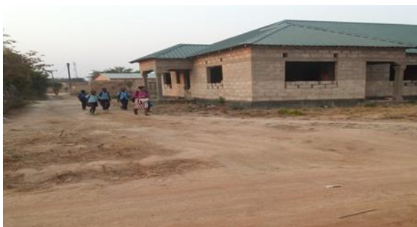
(a) Unfinished house built with concrete blocks.
