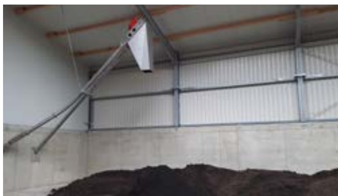
The drained solid matter has a dry matter content of about 30 percent and serves as a high-nutrient fertiliser that is easy to transport.
