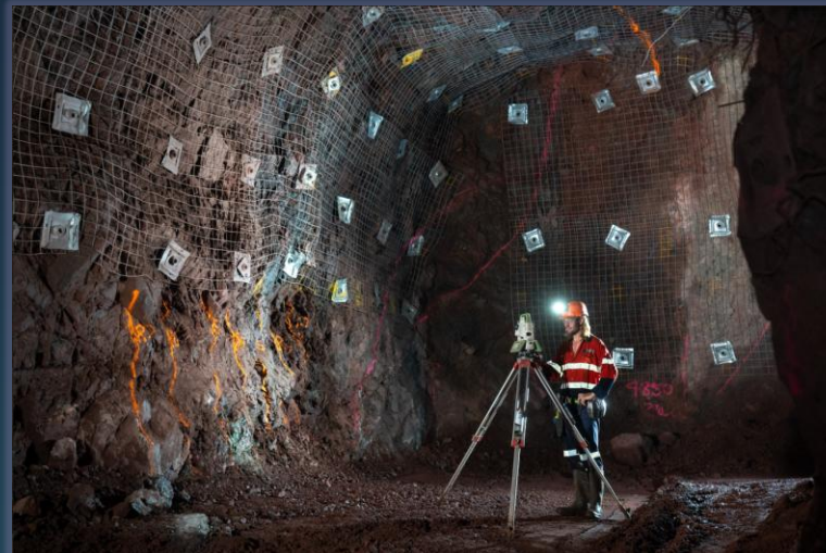
Established underground development
