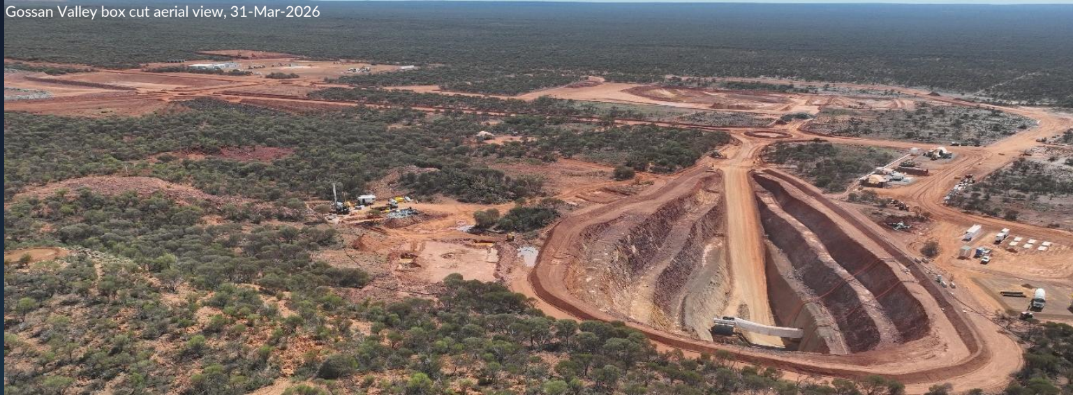
Gossan Valley box cut and decline development - iso looking north-east
