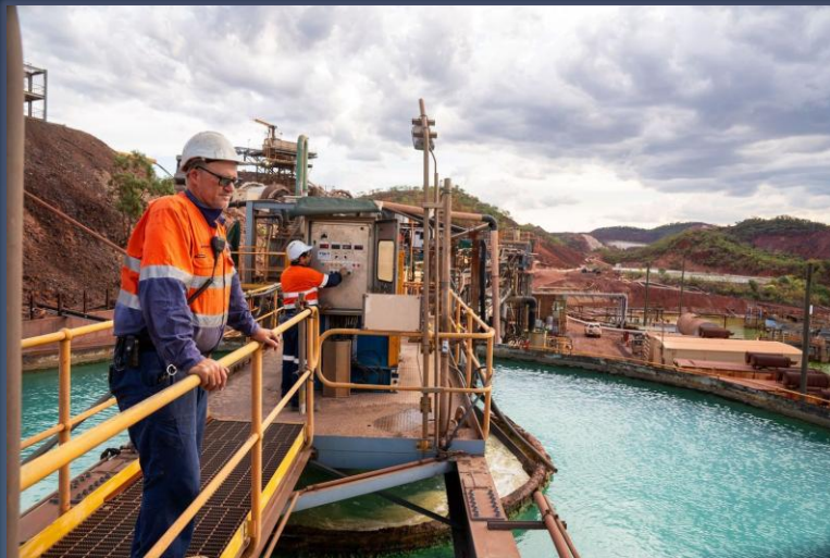
Processing plant & surface infrastructure
