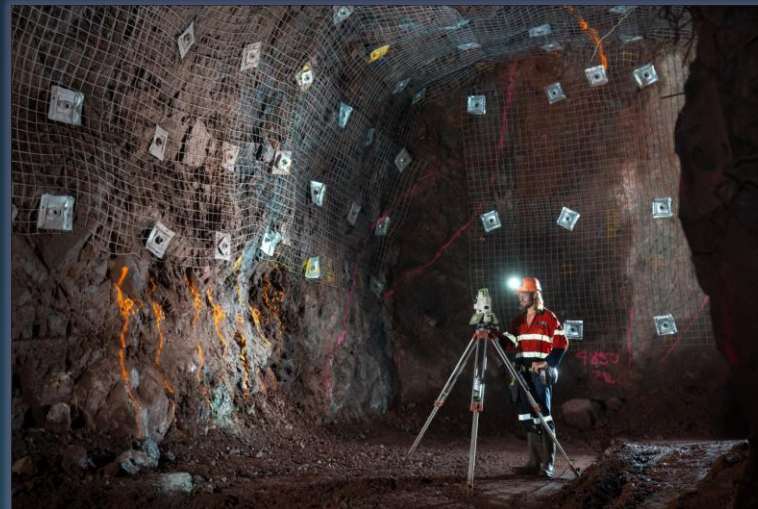
Established underground development
