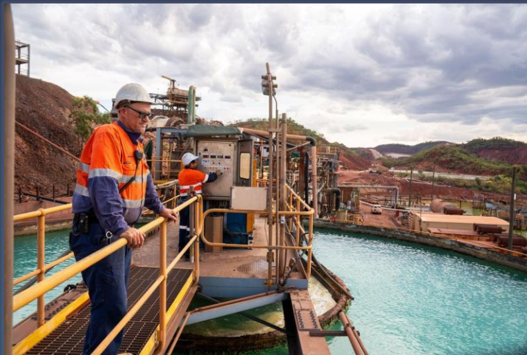
Processing plant & surface infrastructure
