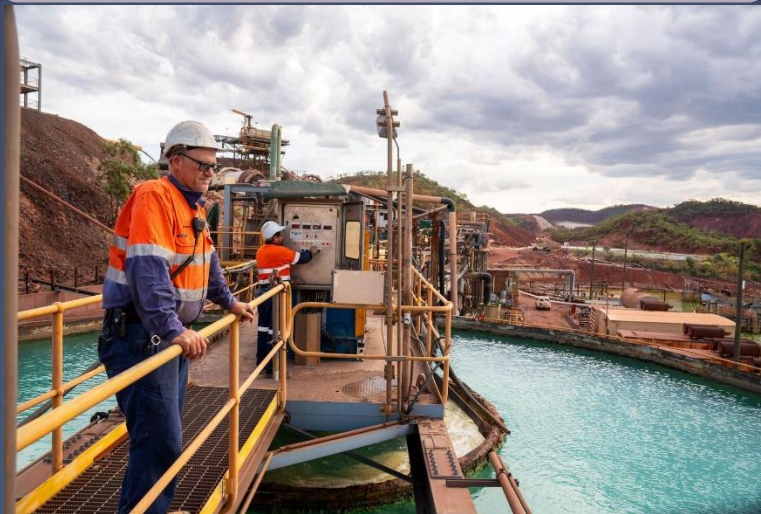
Processing plant & surface infrastructure
