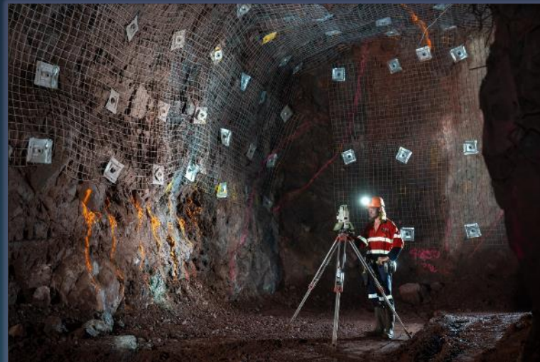
Established underground development
