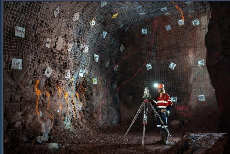
Established underground development
