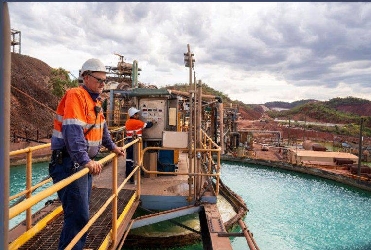
Processing plant & surface infrastructure
