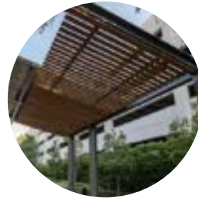
Use light-weight materials for structures to increase shade provision
