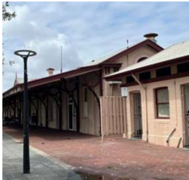
Above: Current state of the Toilet Block, 2025 (Source: Element Advisory)
