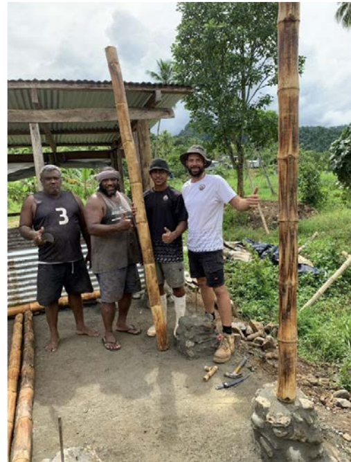
Figure 6-10: Construction of the bamboo market stall at Da Roko Settlement with community participation and hands-on guidance throughout the build by Pacific Ark (Sept 2024)
