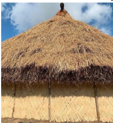
Figure 4-8: Use of bamboo for weaving walls in bure
