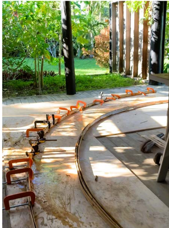
Figure 6-13: Curved prefabricated bamboo beams prepared for the Urata Playground structure by Pacific Ark (July 2025)
