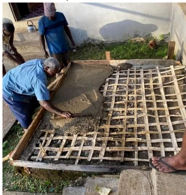
Figure 6-5: Workshop in Nameka village to construct a bamboo-reinforced base for the village bamboo tank by S. Soko
