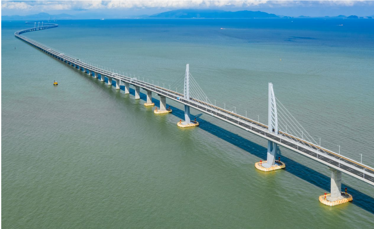
Chinese engineers used bamboo in the world's longest sea bridge 56
