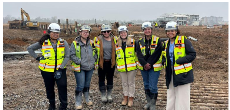
March was Women in Construction Week, but we celebrate the women on our team every day. Their skill and dedication continue to drive the Pimlico Redevelopment project forward.
